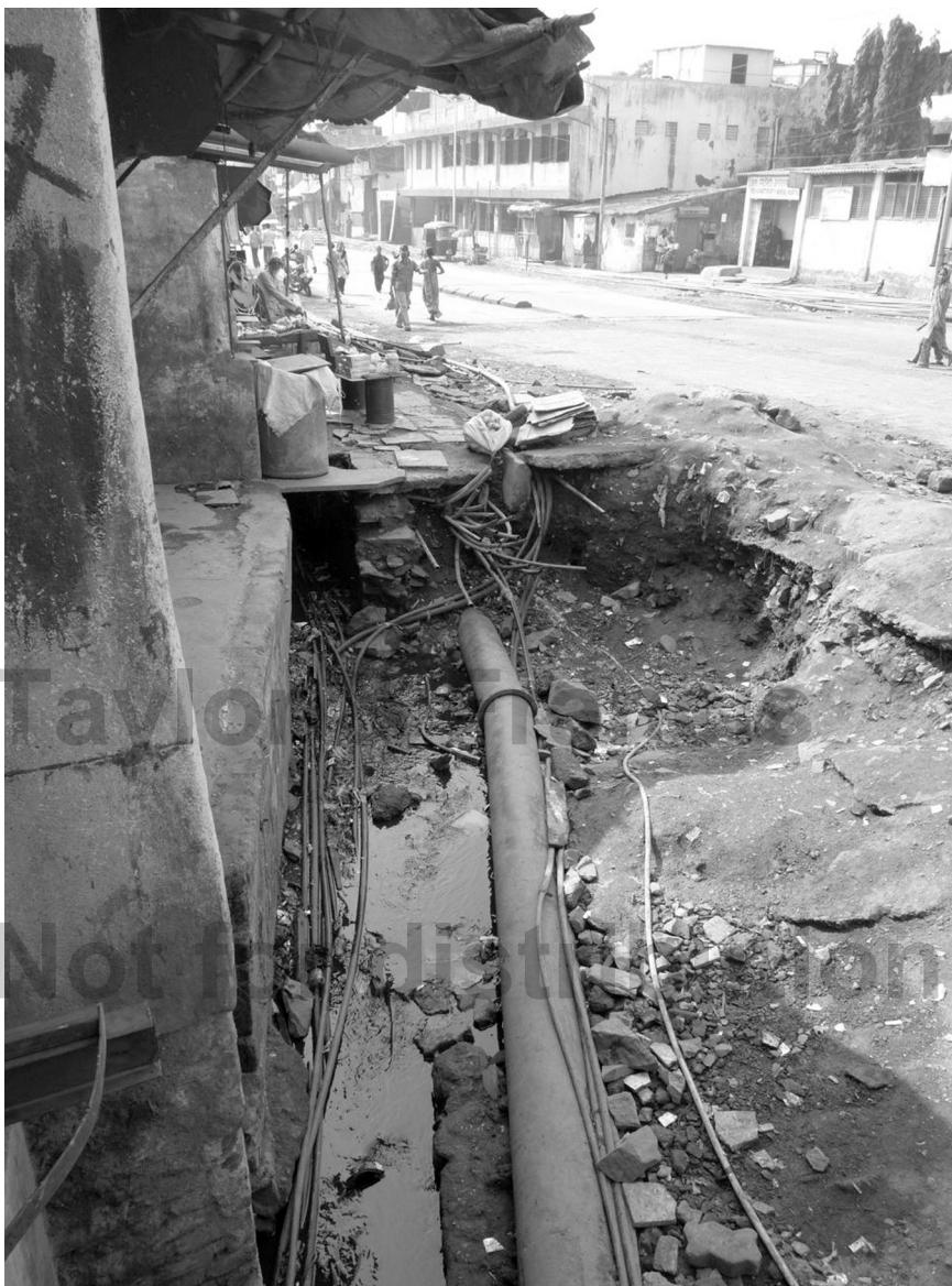
Figure 3.3 Water pipes cut in Rafinagar during the water raids in December 2009
