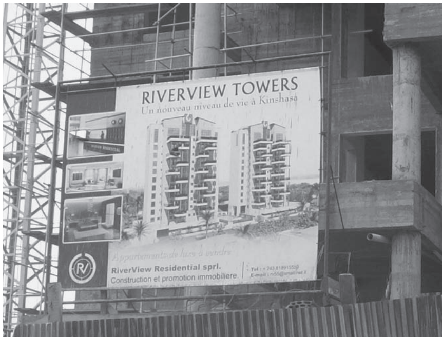
PLATE 19.2 A new level of life: construction in downtown Kinshasa
